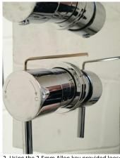
2. Using the 2.5mm Allen key provided loosen the grub screw and remove the Temperature Handle.\*
