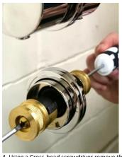
4. Using a Cross-head screwdriver remove the Handle
