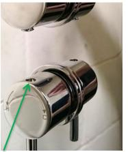
1. Remove the Temperature Handle concealing cap.
