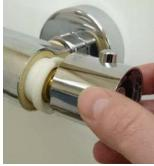
7. Once the Shower is set to the desired temperature, relocate the Temperature Handle onto the Cartridge spline, ensuring that the Over-ride Button Pin is against the Temperature Stop Lug.
