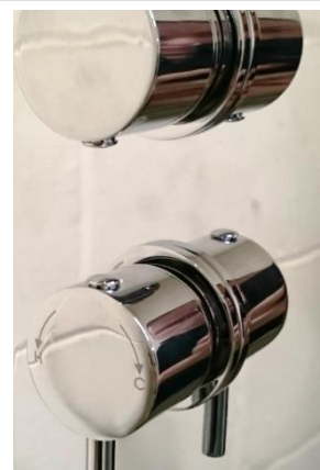
9. Re-fit the Temperature Handle Concealing cap.
