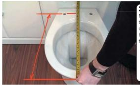
Measure from the fixing hole centres to the front lip of the toilet pan.
