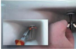
Place the conical washer, stainless steel washer and wing nut onto the threaded bar and tighten. Use pliers to fully tighten the wing nuts.
