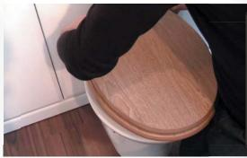
Fit the seat onto the toilet pan and align.
