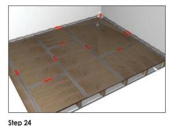
Apply a thin layer of tape sealer to one edge of the floor and adjoining wall approximately 60mm wide on each.
