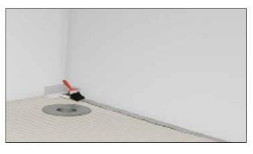
Apply a thin layer of sealing tape adhesive to one edge of the floor and adjoining wall approximately 60mm wide on each.
