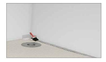
Apply strips of waterproofing tape across all joints and fixing plates using sealing tape adhesive and pressing firmly down. When you have finished you can remove the protective gloves and eye and breathing protection.
