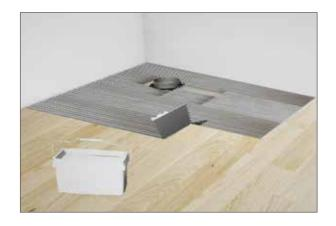
Apply an even thick wavy line of board adhesive across all four edges of the shower tray. Place the shower tray into position and bed down onto the adhesive. Check that the shower tray is level in both directions along the edge using a suitable level.
