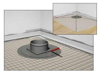
Place the Shower Drain Top face down over the centre of the drain hole then mark around it with a pencil. Mark a line from each of the four corners of the drain top to each corresponding corner of the Shower Tray,
