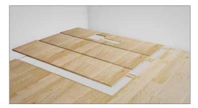
Make sure that the remaining floor boards or sheets in the rest of the room are fully secured down and as level and flat as possible.
