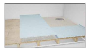
Place the waterproofing internal corners into position and mark around them with a pencil. Once you have marked they can be removed. This is to show where you need to apply the sealing tape adhesive.
