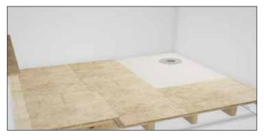
Measure, cut with a safety blade then lay Waterproof Matting in strips to cover the remainder of the floor area around the shower tray allowing a 50mm overlap over the Waterproof Matting strips and 50mm up the edges of each wall. Also allow a 50mm overlap over the shower tray edges. Set the strips of Waterproof Matting to one side.
