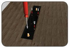
Line up the linear drain bowl with the drain top pre-fitted within the shower tray and connect the two together using the four bolts provided and a suitable cross headed screwdriver.
