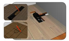
Measure the shower drain base position on the floor and mark this onto the relevant flooring. Using a jigsaw cut a hole in the plywood so that the shower drain base and shower drain connector will be exposed through the new floor.
