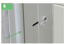
Offer door(s) / fixed panel into their respective compensator ensuring that the slots engage with the adjusting screws. Tighten adjusting screw with the supplied allen key.
