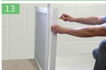
If fitting a post compensator, inline or off a return panel, place the compensator against the post and mark through the fixing slots. Find the centre of your mark and drill a 3.8mm dia hole. Fix in place with No8 x 25mm pan head self tapping screws. Offer door into post compensator as described in steps 4 to 8.
