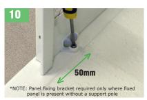
Mark hole through the panel fixing bracket onto the tray or floor & bottom rail (when door and / or fixed panel are inline). Pilot drill and fix bracket in place using self tapping screws and grey caps provided.
