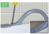
Place door handle(s) against the leading edge of the door(s) on the top rail. Using a 3.0mm drill bit, pilot drill the top rail and fix handle to the door with the countersunk self tapping screws. Fit blanking caps, see inset image.
