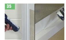
**IMPORTANT:** Seal all joints between compensators, walls, panels and shower tray or floor, on the inside and outside of the shower area using a waterproof, anti fungal silicone sealant.
