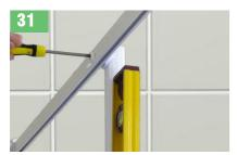
Ensuring the post is straight, pilot drill through both the curtain rail and post using a 3.0mm drill. Screw both together with a No8 x 38mm pan head screw and cap.
