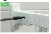
Place curtain rail into wall brackets. Mark holes onto curtain rail through wall bracket on both sides and pilot drill rail with a 4.5mm diameter drill.
