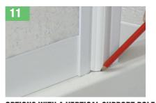
**OPTIONS WITH A VERTICAL SUPPORT POLE:** Insert the panel in the compensator as Step 4, mark around the post(s) to ascertain the location for the post block(s) when the panels are in the correct position.
