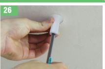
Mark position for the ceiling rose and fix to the ceiling using a suitable fixing (not supplied). Cut drop rod to length.
