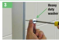
Drill holes in the wall with a No10 masonry drill bit, insert wall plugs, and fix with the No8 x 50mm pan head wood screws and heavy duty washers provided.
