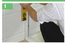
Place compensators against the wall ensuring that they rest on the flat area of the tray or floor at the position shown. Mark off fixing holes on the wall when level.
