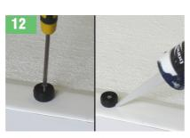
Find the centre point for the post block(s), pilot drill a 3mm hole. Fix block in position with a No8 x 25mm pan head screw. Use a small amount of silicone sealant around the post block(s) and re-fit panel assemblies in position. Fully tighten compensator adjusting screws to secure in position, as **Step 9**.
