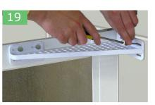
Place panel support bracket against wall and just below the top edge of the top rail (Approx 5mm), on the inside of the enclosure. Mark & pilot drill holes on the rail & wall and fix the bracket in position with the supplied screws and cover caps.
