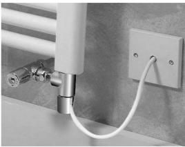
As shown above elements must be installed in the bottom of the radiator either horizontally or vertically.
