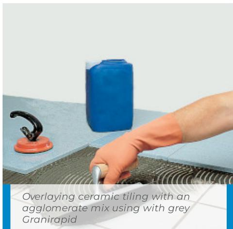
*Overlaying ceramic tiling with an agglomerate mix using with grey Granirapid*
