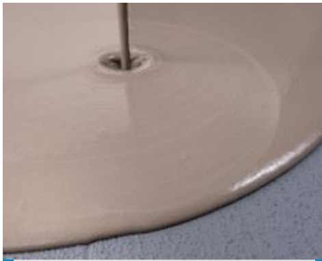
Application of self-levelling smoothing compound on dry Eco Prim Grip Plus on old floor
