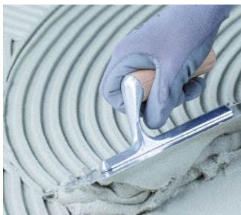
Spreading Adesilex P9 white
