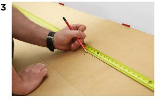
Measure from wall to wall and ensure that you start installing in a logical place to minimise any cut planks to the perimeter of the installation. Mark a "starting line" on the floor with your pencil. Ensure that you include the 5mm expansion gap when measuring. More information in the detailed fitting instructions in each box.
