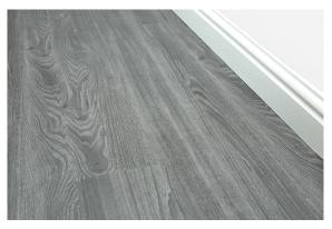
Now your floor is fully installed, you can replace your skirting boards. Be careful not to fully trap the flooring as it needs to be able to expand and contract freely. Usually 1-2mm is enough to allow this to happen. If you left the skirting boards on, then use Scotia beading to cover your 5mm expansion gap. Never use any type of filler to cover your expansion gap.
