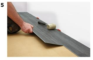
Start the installation by angling each plank into the click locking system along the long ends and then lay each plank flat to the floor. The long ends have a click lock system to hold each plank in place. The short ends have a drop lock system.
