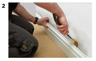
A 5mm expansion gap is needed around the entire perimeter of the flooring. You may wish to remove the skirting boards and replace after installation or use Scotia beading to cover the expansion gap. In this instance we have removed the skirting boards.
