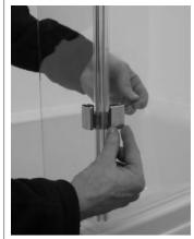
FIT LONG BOTTOM SEAL to front panel glass ensuring 18 that the factory fitted end grommet is pushed fully up to the tube.
