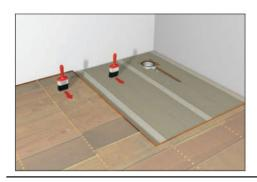
Lay the shower tray into the required position to check the fit of the shower drain base. Once you are happy with the fit, carefully remove the shower tray and store somewhere safe.
