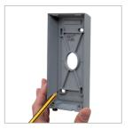
Drill and prepare the wall fixings for the controller using the fixings provided, if suitable.
