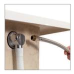
Connect the flexible hose to the blended supply pipe ensuring suitable non restrictive double check valves are fitted in line with current Water Supply Regulations (not supplied).
