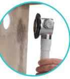
Ensuring the rubber washer is correctly aligned, pass the overflow filler outlet through the bath and secure to the body assembly.
