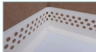
9. Ensure that the seal is not stretched too tightly at the corner. It is very important that when placed in position, the seal fits neatly into the corner of the supporting walls. **If it is too tight, this could compromise the seal, and make tiling difficult.**
