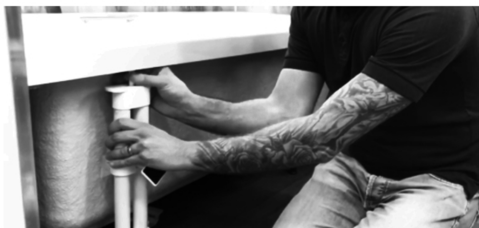
Place circular pad under bath lip and tighten
