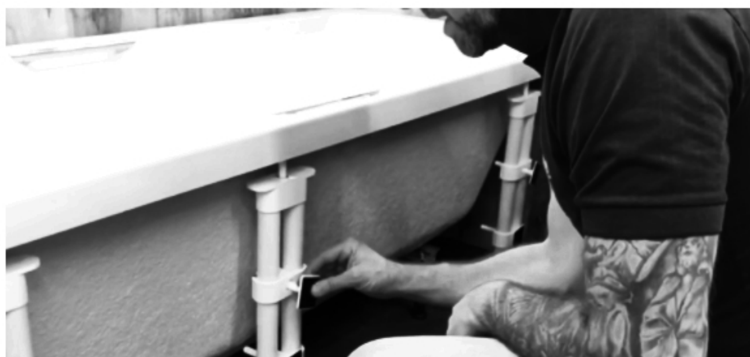
Threads can be cut shorter for narrow bath edges
