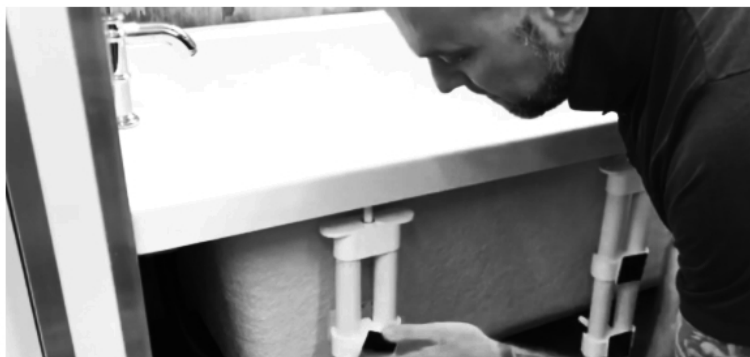
Screw in shortened threads
