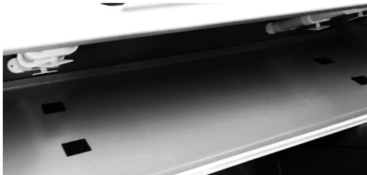
Apply opposite velcro pads to the bath panel
